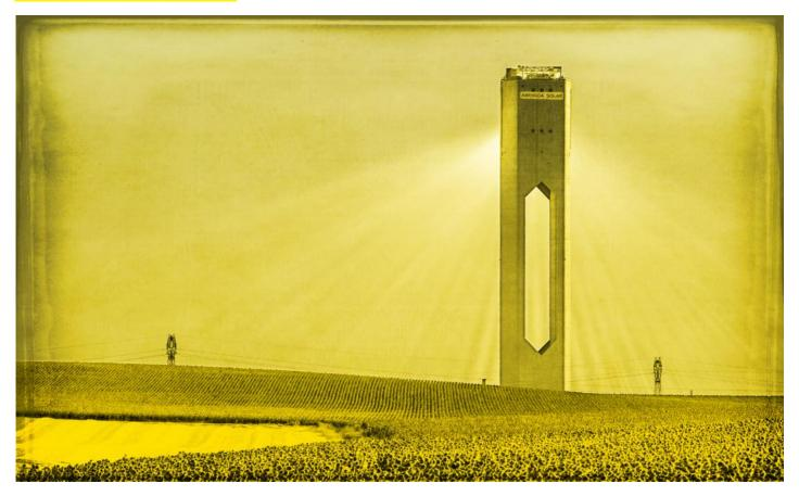
The solar power tower technology involves capturing solar radiation using dual-axis mirrors that track the sun, and reflect sunlight onto the receivers. The solar power plant Planta Solar 20 can power about 10,000 homes.
