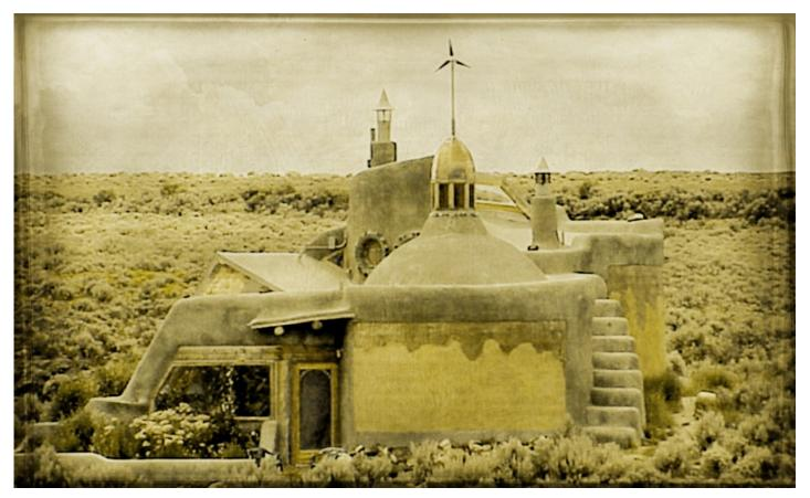
An Earthship is a type of passive solar house that is made of both natural and recycled materials such as earth-filled tires. Earthships are intended to be off-the-grid ready homes with minimal reliance on both public utilities and fossil fuels.
