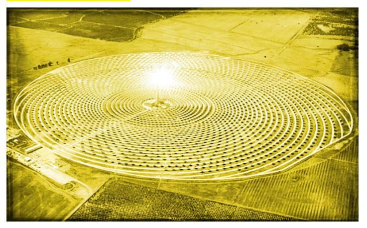
The Gemasolar power plant can store heat to power turbines for 15 hours without exposure to sunlight. Therefore the plant can generate electricity also in the night. The plant is surrounded by 2,600 mirrors and is located in Seville, Spain.
