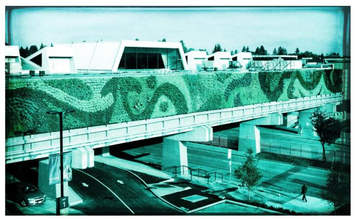
Living walls are self sufficient vertical gardens that are attached to the exterior or interior of a building. The living installation works to draw pollutants and CO2 from the air and returns fresh oxygen and moisture.
